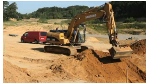
Image 5: Ditching the pit
