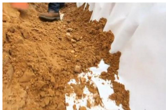
Image 11: Backfilling filter fabric for fixing
