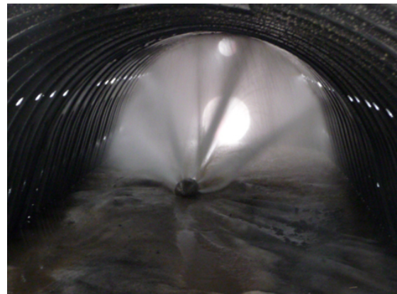
Image 15: High pressure cleaning
