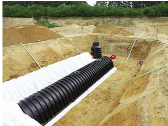
Image 10: Covering with filter fabric
