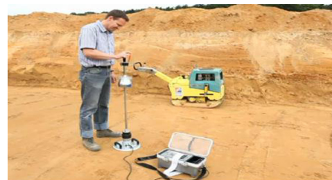
Image 6: dyn. Plate load test at ground level
