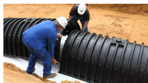
Image 9: Form lock fixing of two tun-
