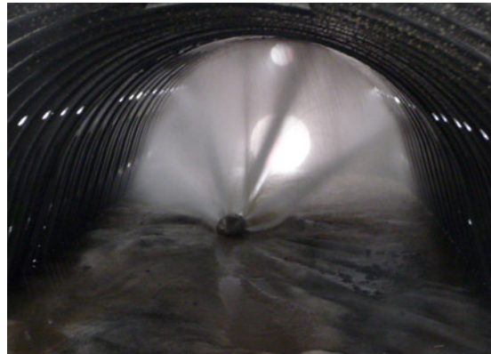
Image 4: Flushing nozzle with cleaning procedure
