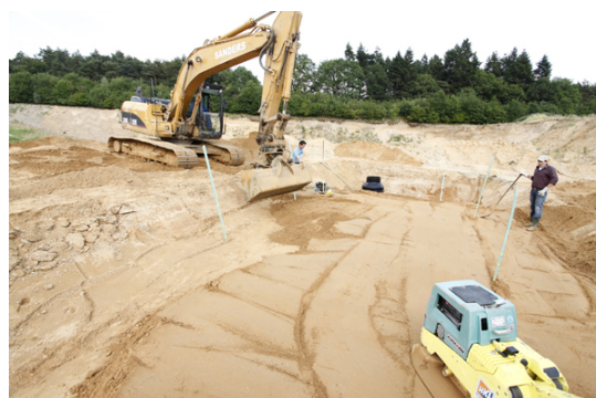
Image 13: Covering the tunnel elements
