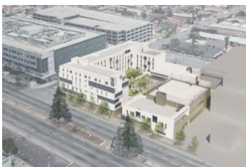
School in LA in the USA
