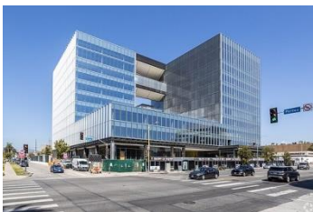
Lumen Office Campus in the USA
