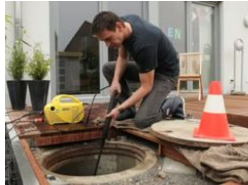
Fig. 15: Cleaning the surface of sieve with high pressure cleaner
