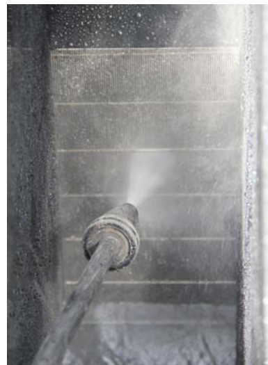
Fig. 16: Automatic cleaning with high pressure cleaner
